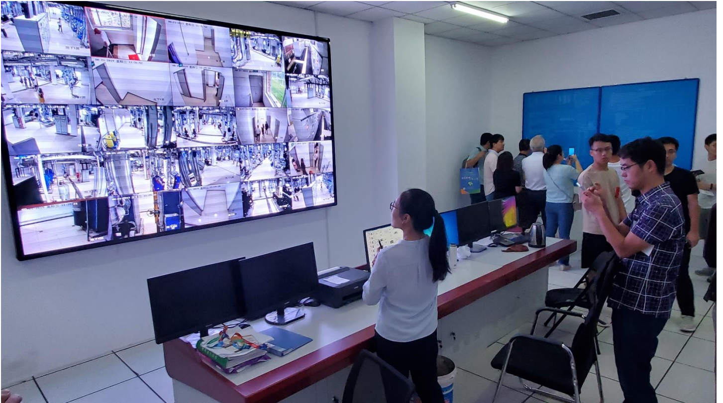
Monitoring the geothermal system.
